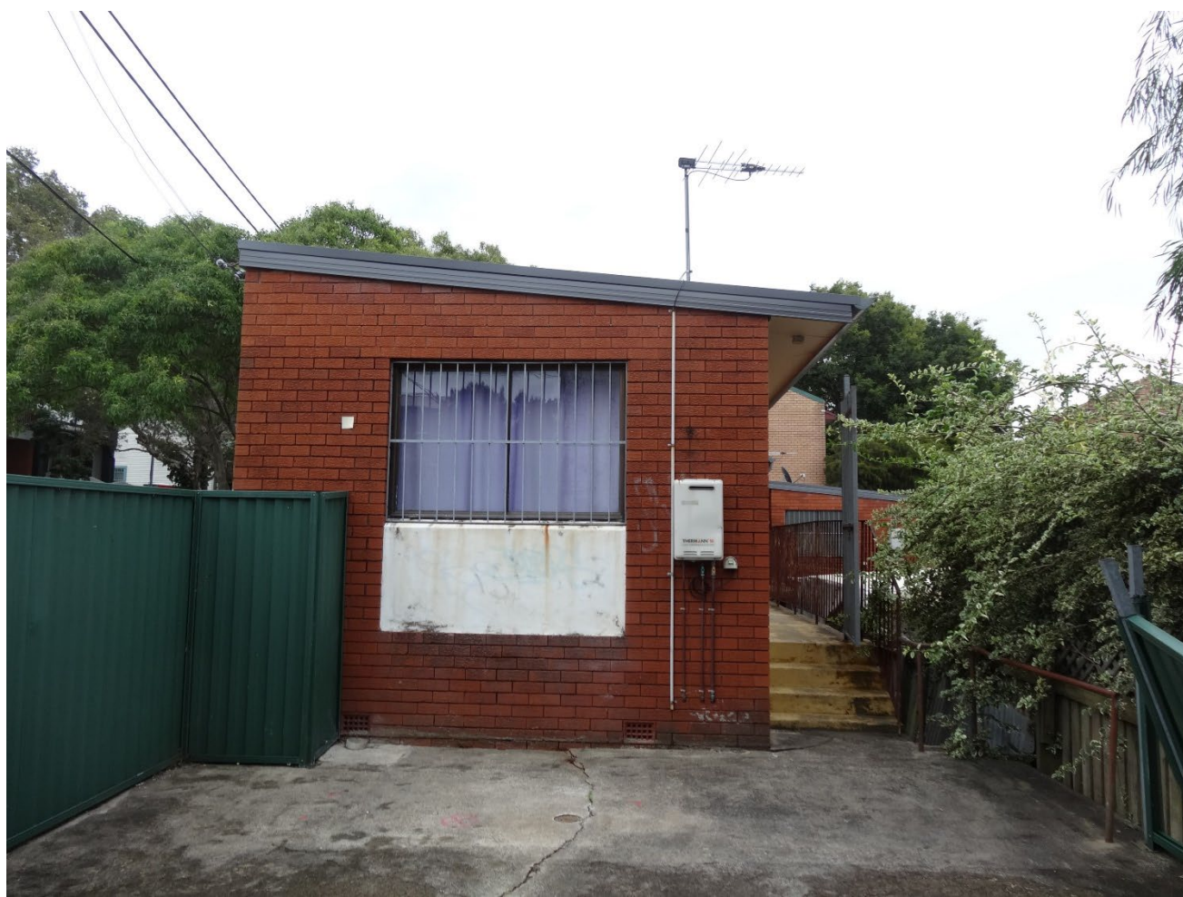
view from existing hardstand (east side of building)
