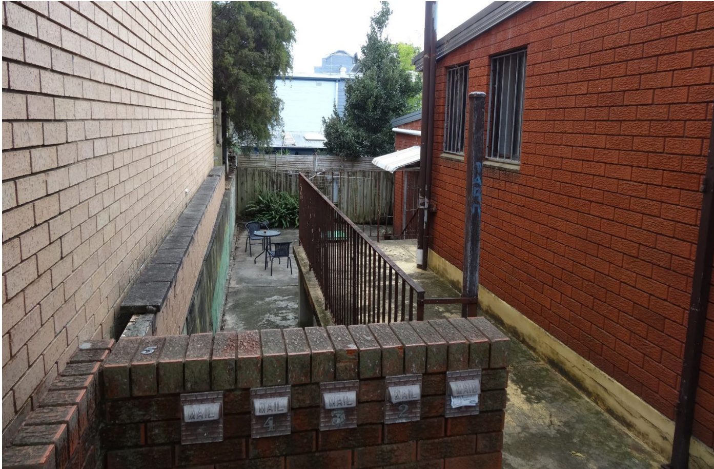
side passage adjacent to 30-40 Bray Street (west side of building)
